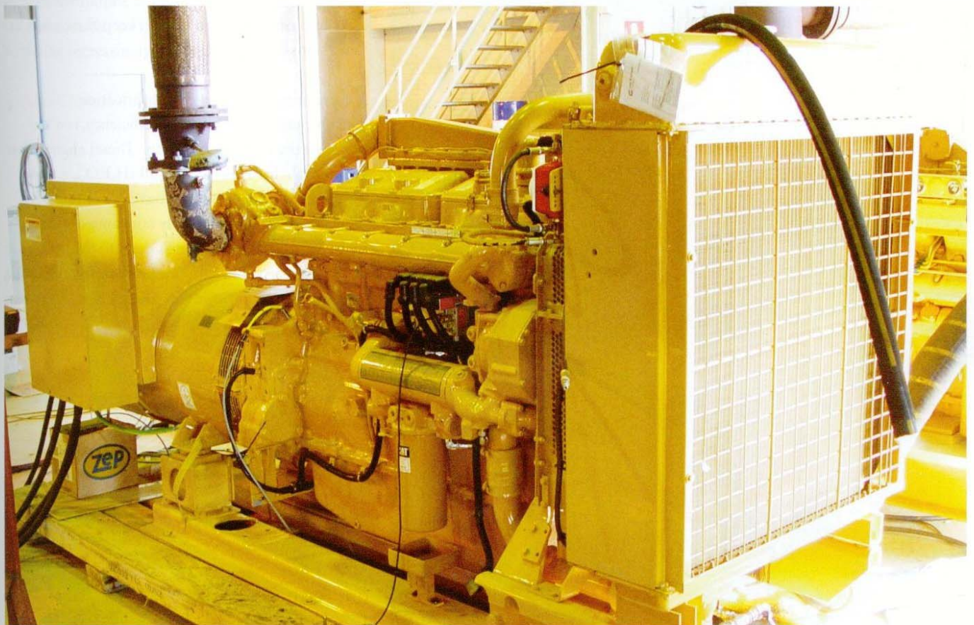
▼ A high-speed four-stroke in-line engine with radiator cooling for a generator.
