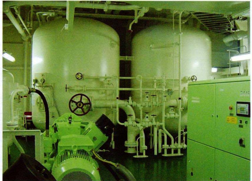
▲ The air receivers for a large two-stroke crosshead engine – Category IV.
