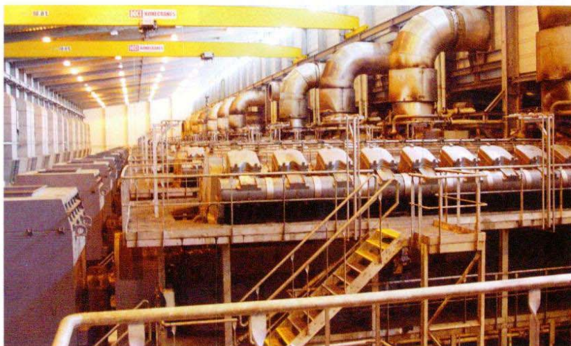
▲ Fourteen eighteen-cylinder MAN-B&W – V-48/60 type A&B diesel engines in a diesel-electric power plant in San Pedro Sula, Honduras, Central America.
