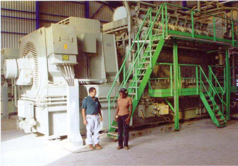
◀ A four-stroke medium-speed Deutz 640 diesel engine for H.F.O. in a diesel power plant in the Gambia.
